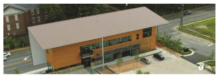
▲ VMZ Double Lock Standing Seam Panels in Pigmento Red from VMZINC were used on the AIA North Carolina chapter building in Raleigh.
