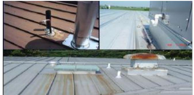
Figure 2. The harmful effects of copper runoff
