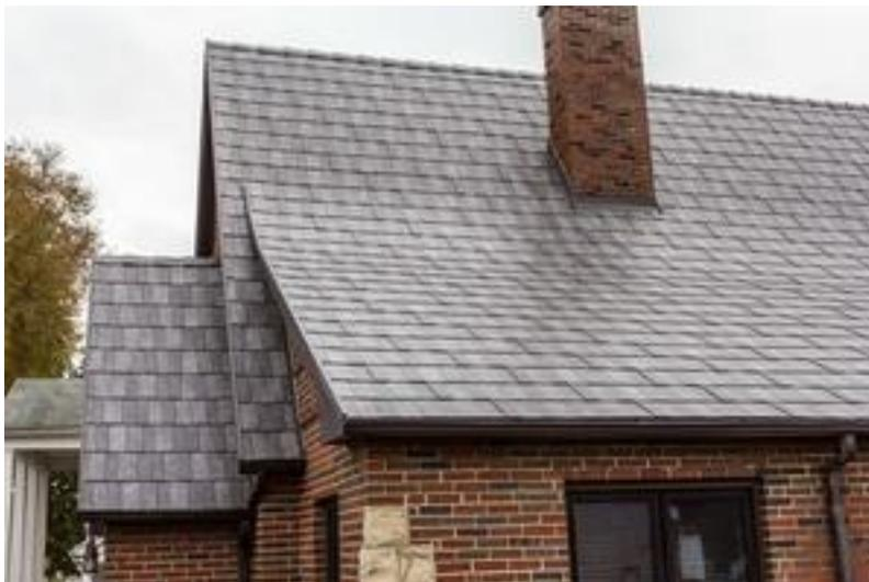
For homeowners who want all of the benefits of a metal roof without the traditional metal roof appearance of a standing seam or exposed fastener system, there are a couple of [specialty metal roofing panel](#) options.
