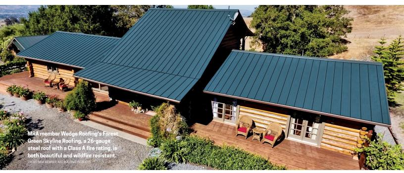
A Class A assembly includes using a fire resistant sheet under the metal, removing the intake for the attic from under the eaves and putting it on top of the roof (to prevent hot attic air from drawing cool air under the eaves up into the attic, spreading the fire), and offering Fire and Ice underlayment that "ooze seals."
